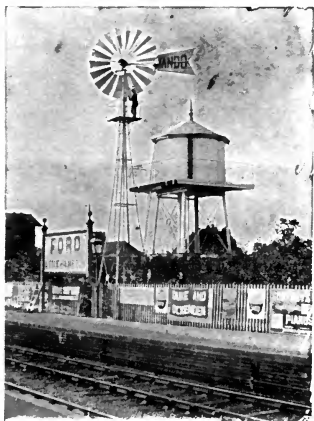
'Dando' Self-regulating Windmill with Reservoir.
