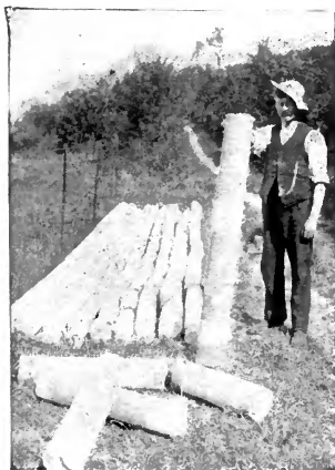
Cores produced by 'Dando' Rotary Driller.
